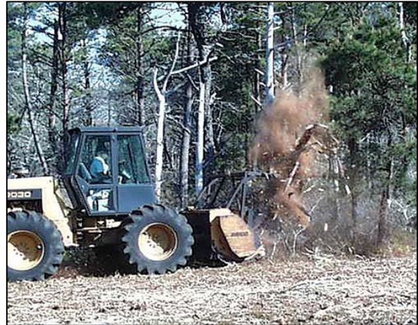
Figure 29: Front end loader with Fecon mastication head Credit: William Patterson III, funded by Joint Fire Science Exchange
