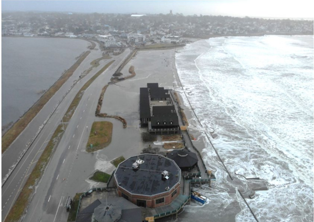
Easton Pond Dam South (left) and Easton's Beach (right) during a storm in December 2023. Photo credit: City of Newport.
