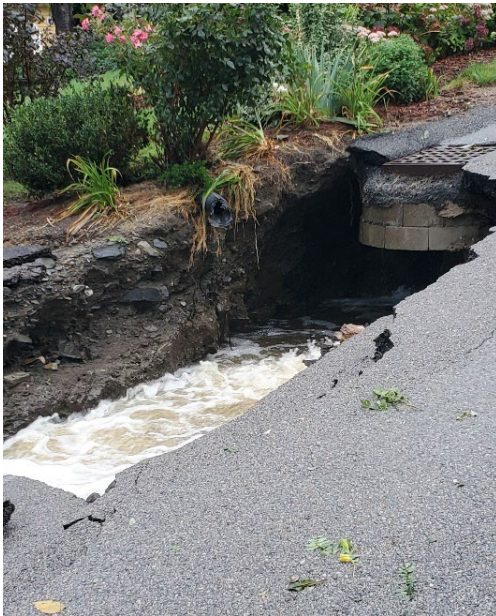
Underground catch basin (left) and road (right) collapsed after heavy rainfall from the remnants of Hurricane Ida in 2021. Photo credit: Portsmouth Police Department.
