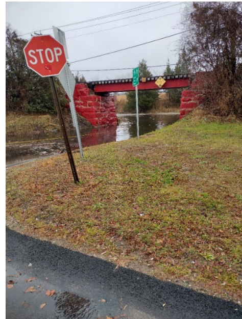
Road flooding at the entrance to Common Fence Point, Portsmouth. Grant money was used to install a better drainage system to reduce the flooding depicted above, but concerns grow as tides creep higher and water egresses in from the drainage system during extreme high-tide events.
